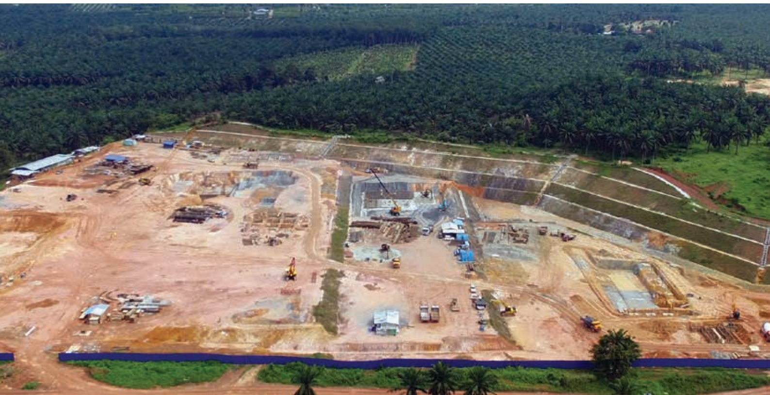
Pagoh Water Treatment Plant - Under Construction (Completion Date: 25 August 2019)
